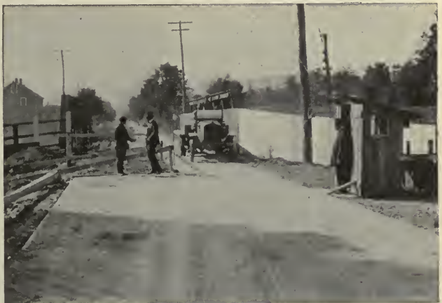
WHEN THE HALF-AT-A-TIME METHOD PERMITS ONLY ONE LINE OF TRAFFIC, THIS IS REGULATED BY A TELEPHONE, IN MASSACHUSETTS
